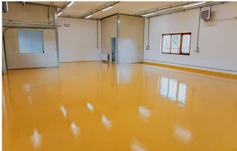
Qinhuangdao Electricity Protection Laboratory, China
