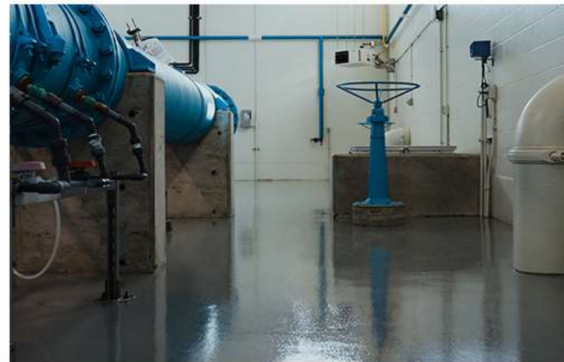
Brooklyn Center, Water Treatment Plant
